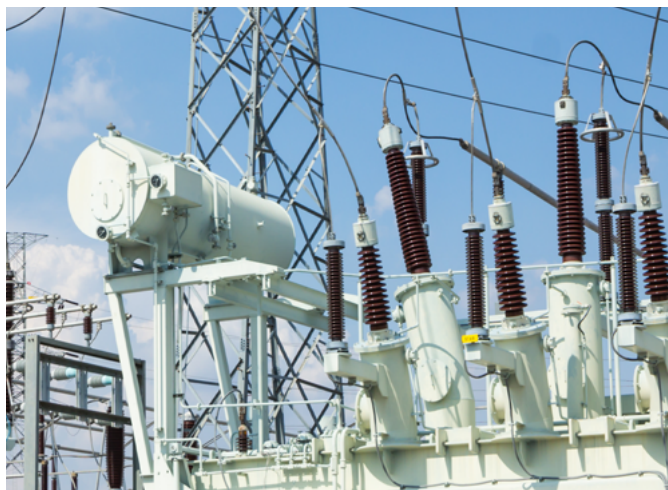
Transformers are critical parts relying on battery backup.
